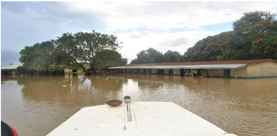
Flooded primary school building
